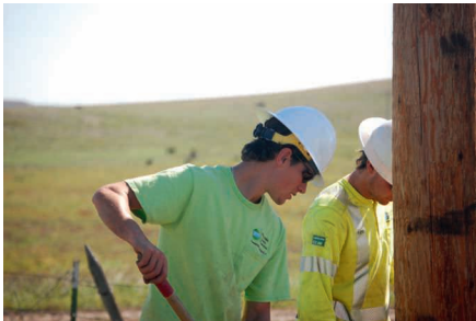
Gavyn setting a pole for new service.
