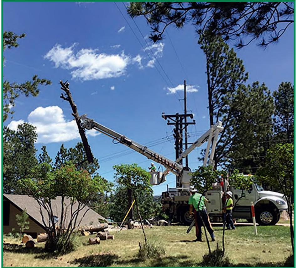
**After using a bucket truck to limb this tree, BHEC's crews used a digger truck to carefully lift part of the trunk over the homeowner's roof. BHEC's rights-of-way program has helped reduce outages caused by trees that are in danger of making contact with the lines. Please contact the co-op if you see a danger tree.**
