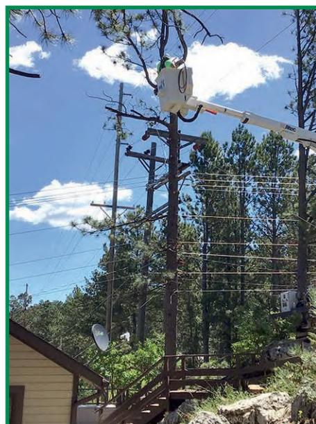
**A maze of wires surrounded this tree that was recently removed by co-op crews. The job required a bucket truck and digger truck to safely remove it.**
